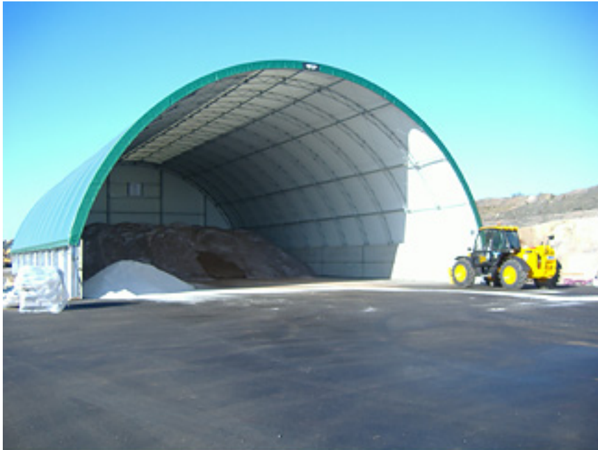
Photograph 2 – Typical Salt Barn, supplied by Peacock, costs £200k for 2000t or £275k for 3000t
